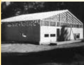
Construction begins in Sooke
